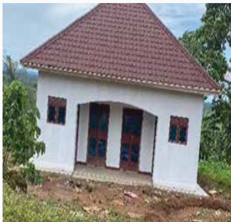
Newly Constructed Midwives House
