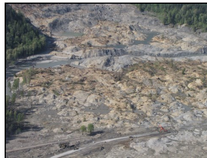
Oso Landslide Blocking Highway 530
