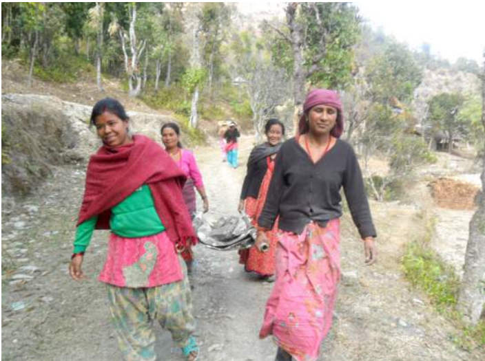
Jagirgaun users transporting local materials to construction site
