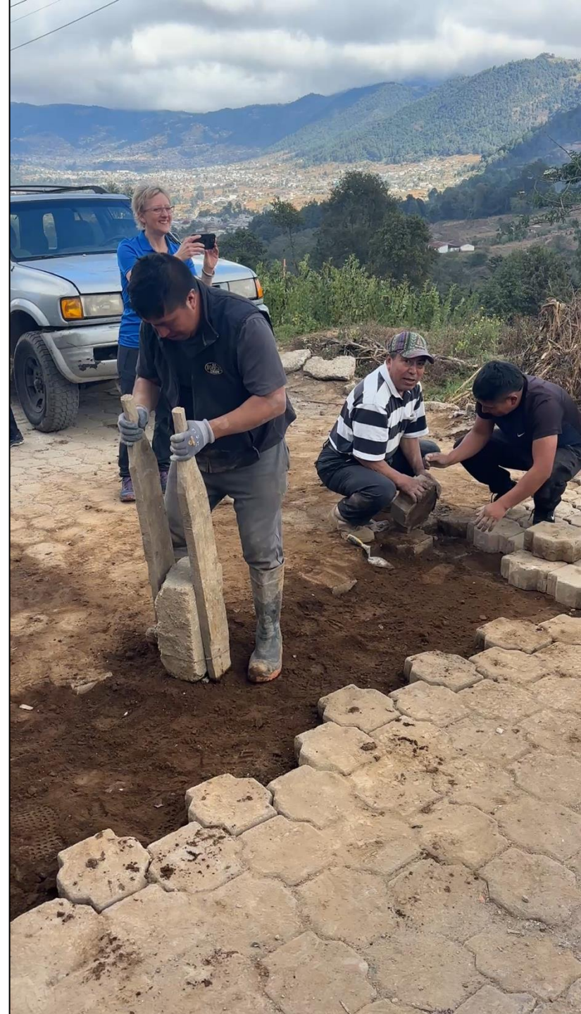
Trench across a road for a feeder line. Then manual repacking of the fill (video)
