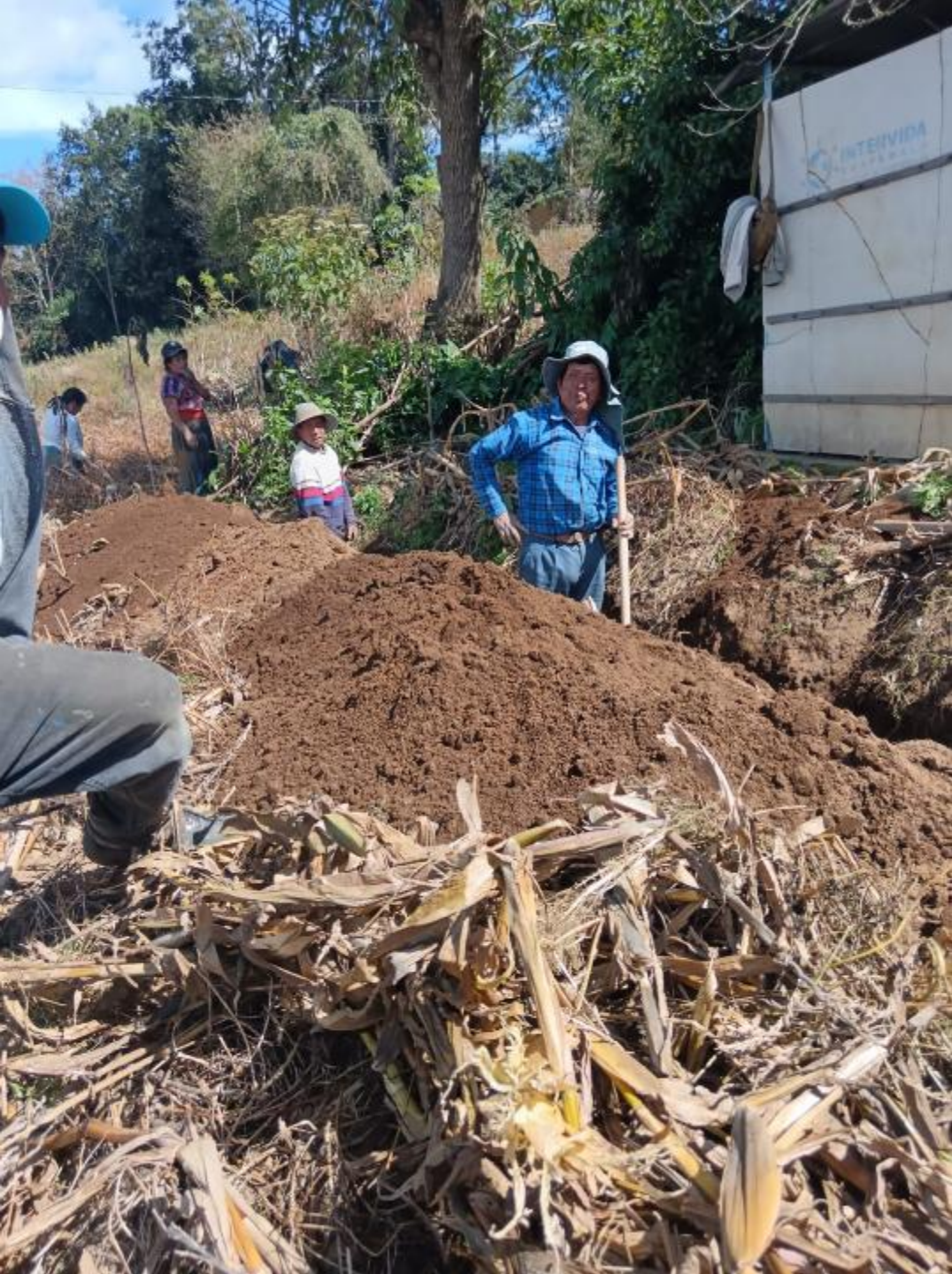
Community members trenching in a corn field
