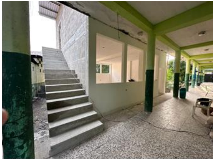
Access from the existing school to the 2 nd level
