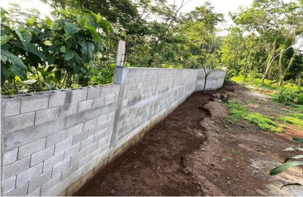
New rear perimeter wall
