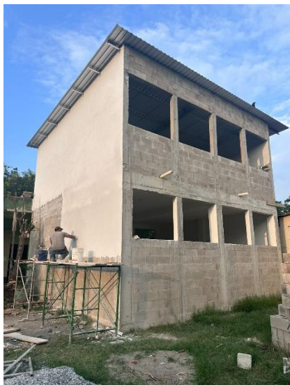
Two classrooms on two levels
