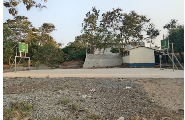
New concrete pad for soccer and basketball
