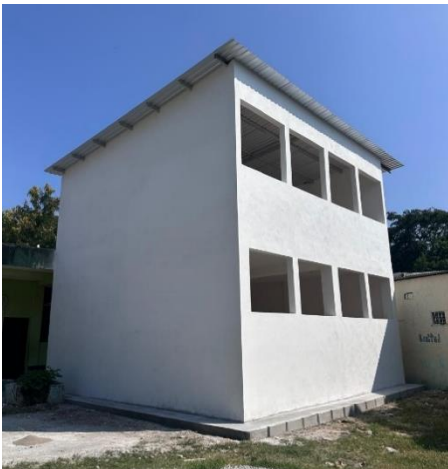
Two classrooms on two levels
