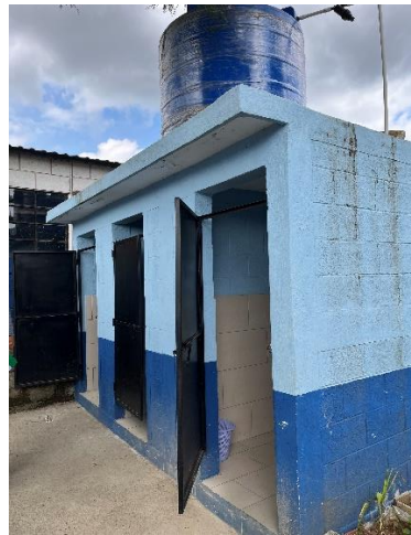
New washrooms and water tank
