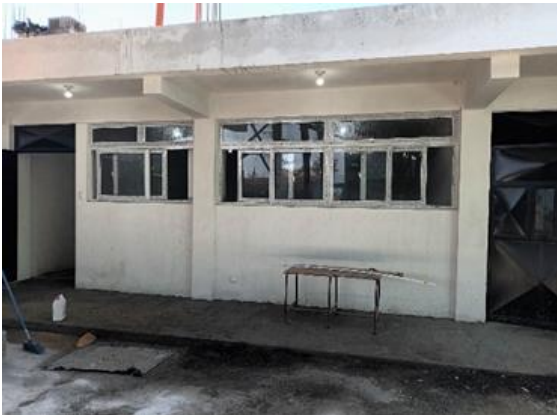
Two classrooms are 95% complete
