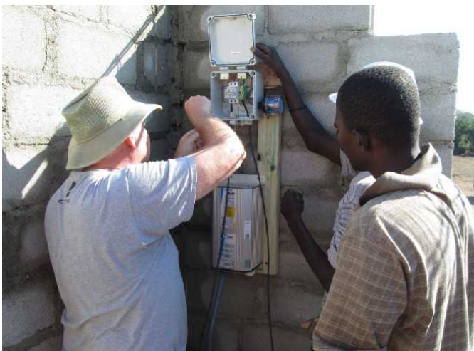
Rick Adams and Haitian Contractor install Pump Controller - January 2016.
