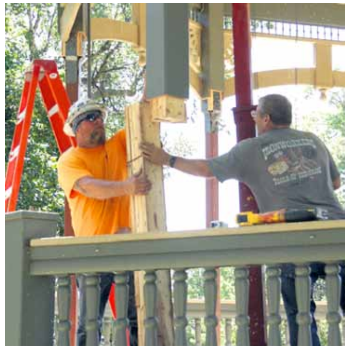
Workers for Seither & Cherry are removing pillars on the Central Park gazebo and putting in metal beams after termites damaged the structure. The pillars will be trimmed to look like wood. Lane Jensen (l) and Mike Johnson are among those working on the project. Democrat Photo by Chris Faulkner
