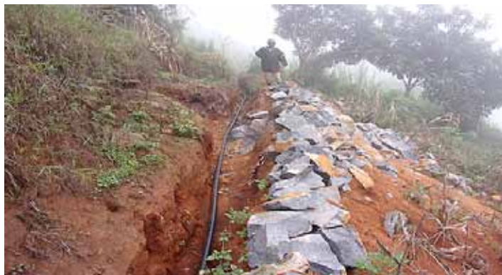
Breaking Underground Rocks to allow trenches for water pipes
