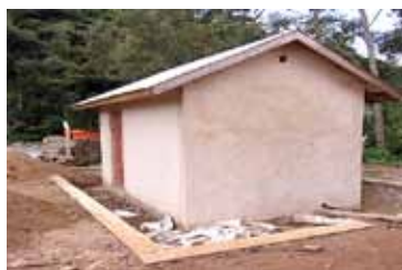
Filtration and treatment house
