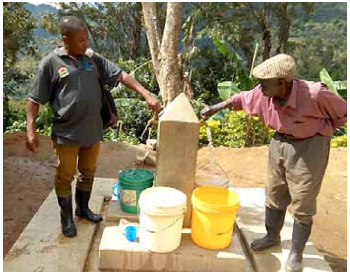
New water distribution point in operation in Mhezi.
