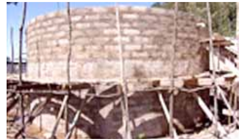
Construction of the water tank.
