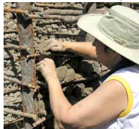
Rachel Litwiller placing mud balls in the wall.
