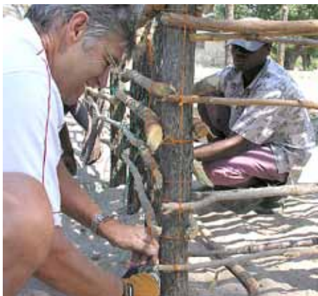
PDG Cal Litwiller tying horizontal twigs to stakes.
