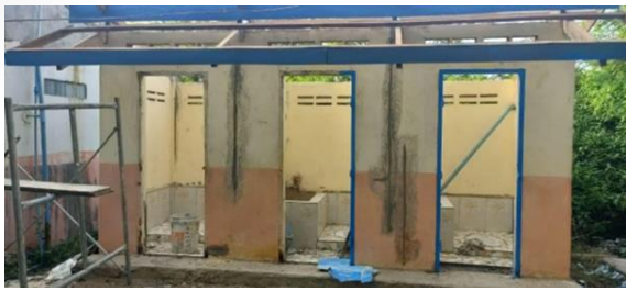
(Renovation of one latrine block, left, and building of the 16-faucet wash area, right)
