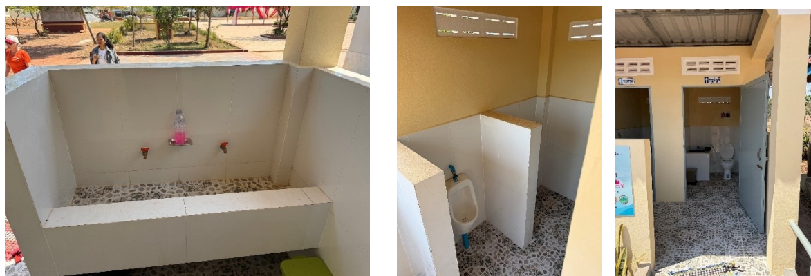
(Overview of the wash area and urinals on the boys' side, and one of the toilets on the girls' side)
