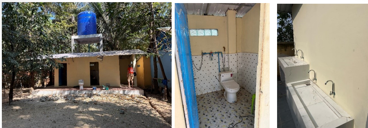
(Finishing touches (top), the completed showers and toilets (middle), and the girls' showers, toilets and a wash area))
