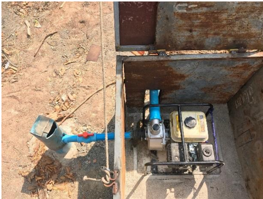
(The well and pump assembly)
