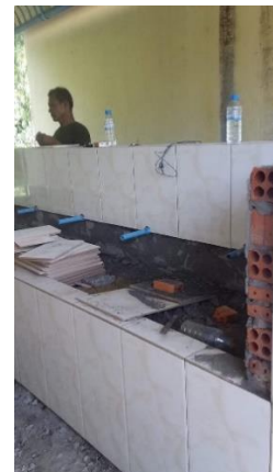
The wash area under construction – the left side has taps for handwashing, while the right side is designed to fill large containers.
