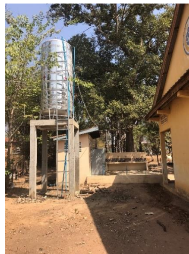
The well and pump assembly (left picture), and the 5000 L storage tank which feeds the latrines, wash areas, and garden. The garden grows various fruits and vegetable for the children's school lunch.
