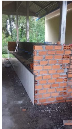
The wash area under construction – the left side has taps for handwashing, while the right side is designed to fill large containers.
