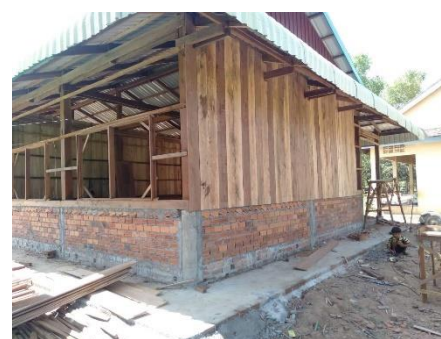
Installing the walls. This project employed up to 10 locals full time for 3 months providing much needed income.
