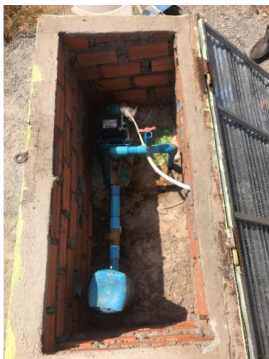
The well and pump assembly (left picture), and the 5000 L storage tank which feeds the latrines, wash areas, and garden. The garden grows various fruits and vegetable for the children's school lunch.
