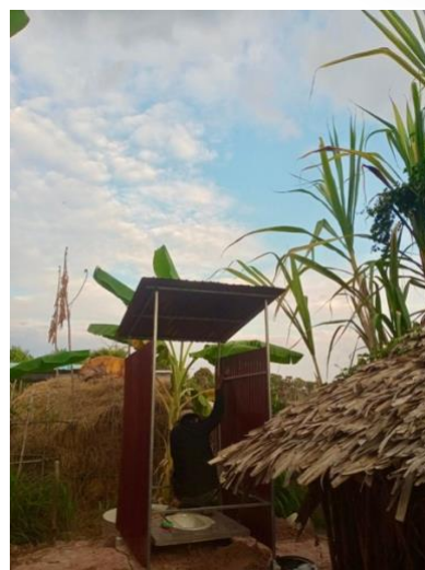
(Local contractors assembling some of the 81 latrines in Siem Reap Province)
