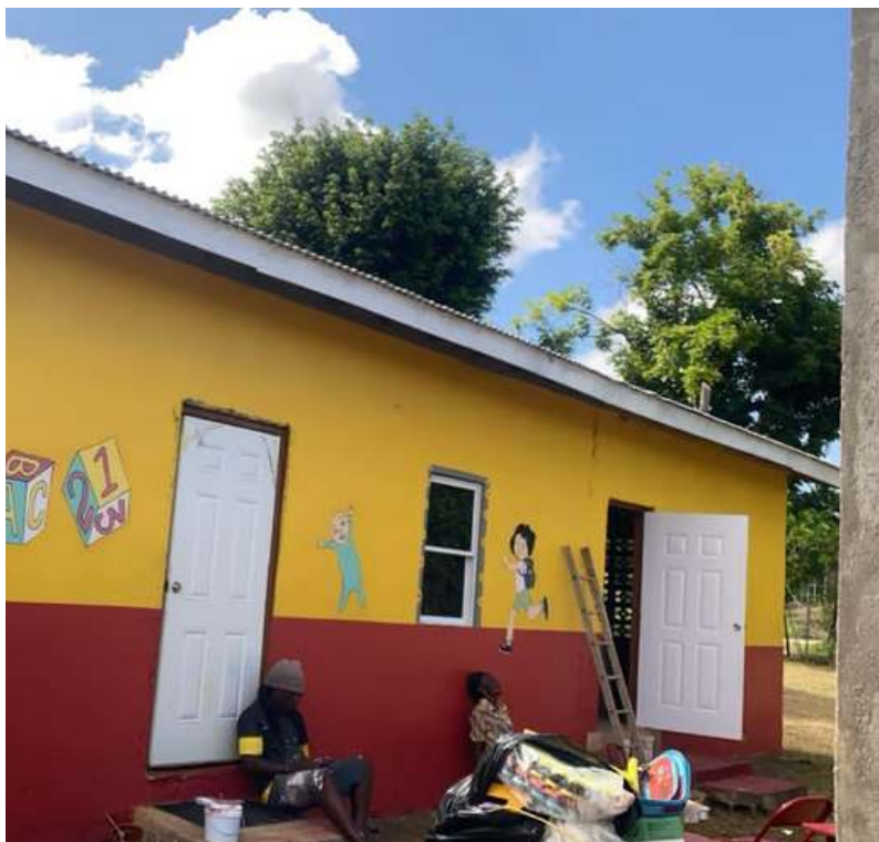
The updating the exterior of the classroom in progress.
