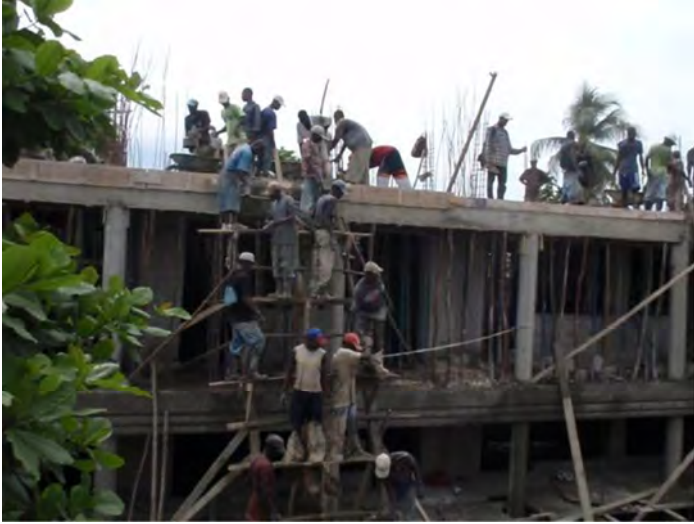
At left - Workers adding concrete to the second roof.
