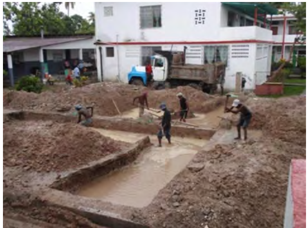
Above – Digging for the foundation of the school.
