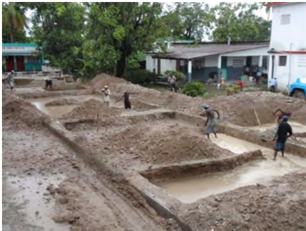
Above – Digging for the foundation of the school.
