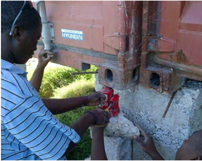
Left – levelling containers - Right – Roof begun
