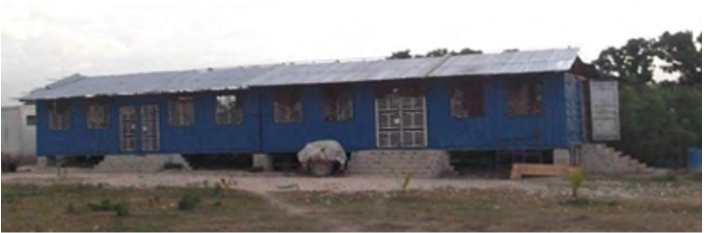
Roof is on
