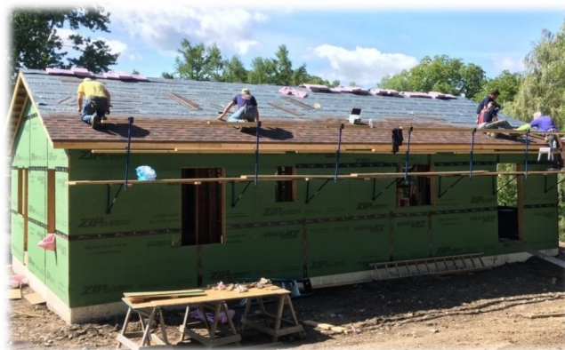
Shingling the 1,200 sq foot, 2 bedroom, 1 bath, new house. First of two being built
