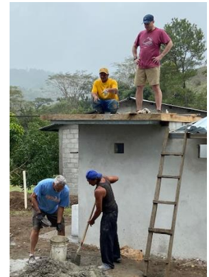
Steve & Jason mixing concrete for the pad on the roof for the cistern
