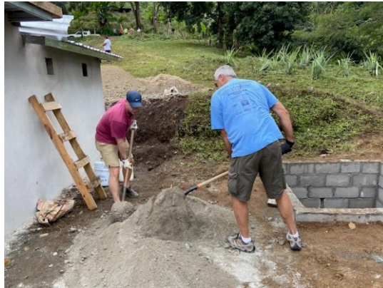
Steve & Jason mixing concrete for the pad on the roof for the cistern
