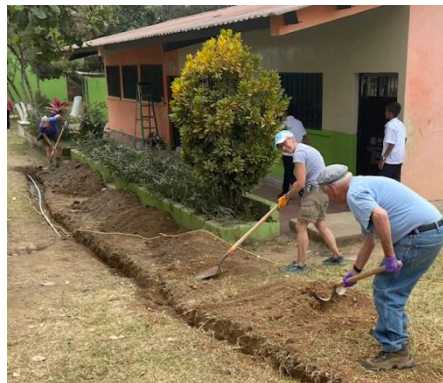
Tosh and Jim digging a water line
