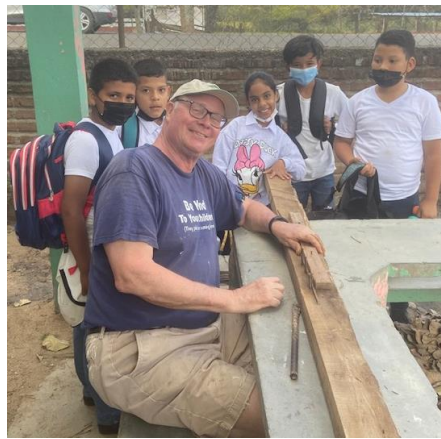
Dave working on Rebar And Attracting the Ninos y Ninas
