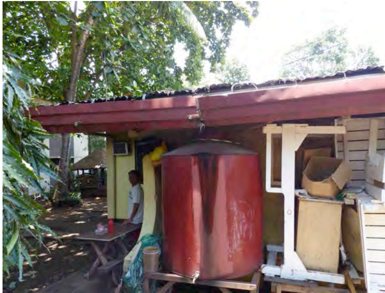
Original water catchment tank and damaged gutters at the House of Hope
