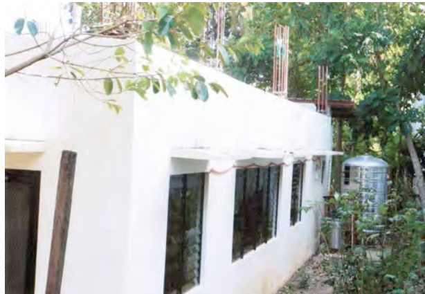
House of Hope Annex with the SS Water Tank and Pressure Pump
