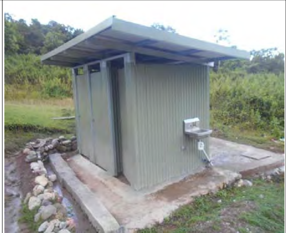
Toilets and more toilets. One down three to go.
