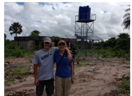
Corey Spies, Dr Brianna Parsons on site. In the background is the finished borehole well which is completely solar powered with capacity to provide the future dairy with 30,000 L of water
