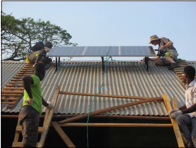
Installing solar panels on the Administration building roof.
