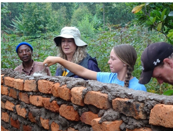
Building Brick walls for a latrine
