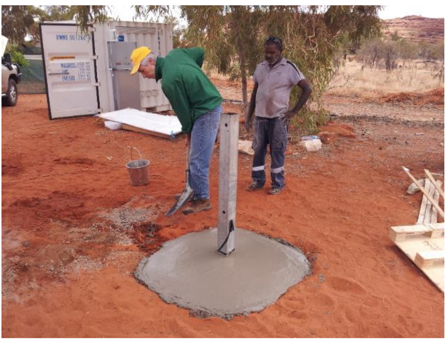
Pouring complete. Photo: Nick Tyllis
