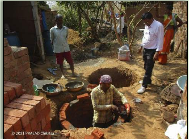
Toilet at Brick Masonry Stage
