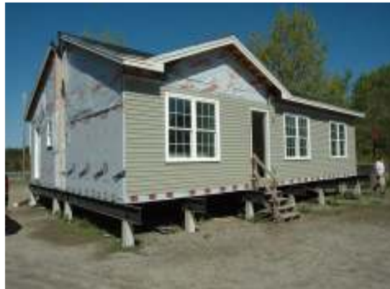
The 2008-2009 almost completed house.
