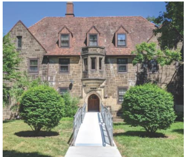
Pictured: New Nielsen House on Millbank St. .
