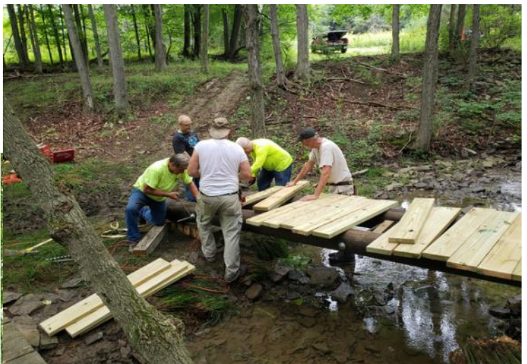
A new 20' bridge with railings was built to replace an old 12' footbridge that was falling into the creek. (l-r) Tyler Smith and DeLos Blackwell, Rotarians Karl Schweisinger and Matt Weibel, and Matt Smith are in the process of installing new treads to the stringers.
