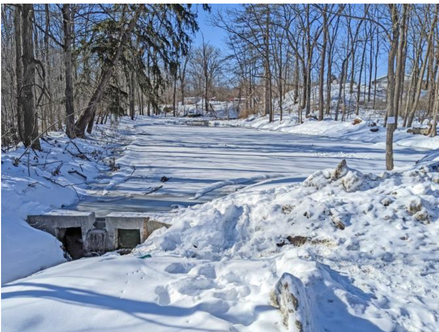
Close up of the weir and sluiceway with some very cold water continuing to cascade over the edge. For some idea of scale and depth, the windows are nominal 2' X 2' squares.
