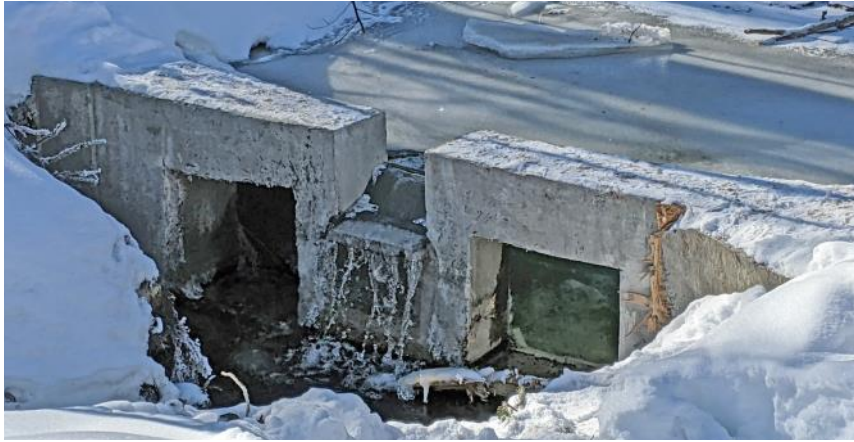
Close up of the weir and sluiceway with some very cold water continuing to cascade over the edge. For some idea of scale and depth, the windows are nominal 2' X 2' squares.
