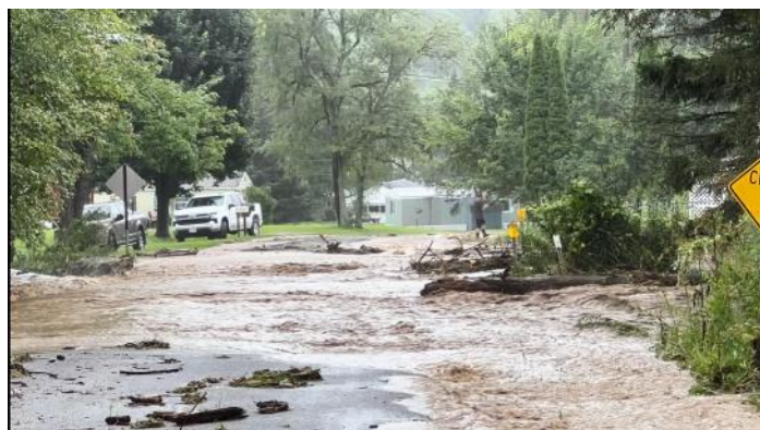
Gary Drum of the Evening Tribune captured this picture of the remnants of Tropical Storm Debby causing major flooding on August 9 th in Southern Steuben County, including the Village of Canisteo.
