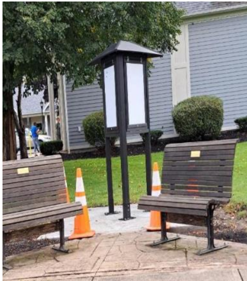
INSTALLED KIOSK SEPTEMBER 28, 2024
