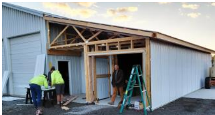
The new Loan Closet building under construction during the fall of 2025. One wall of the structure was an outer wall of one of the Village's DPW buildings.
