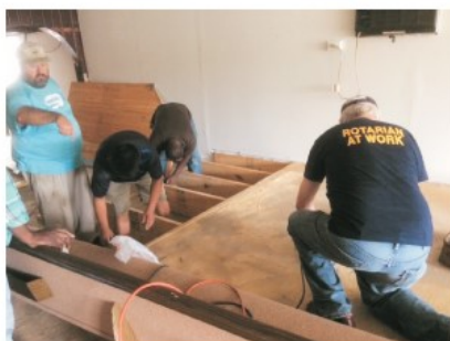
Removing the floor deck
