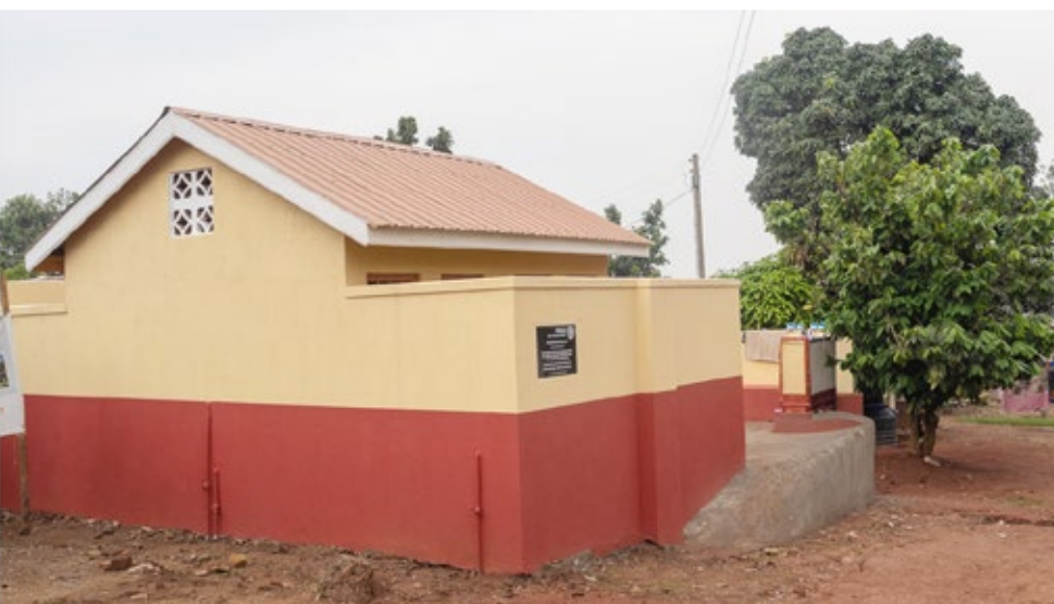
Above: The area before the bathroom was constructed. Below: After completion.
