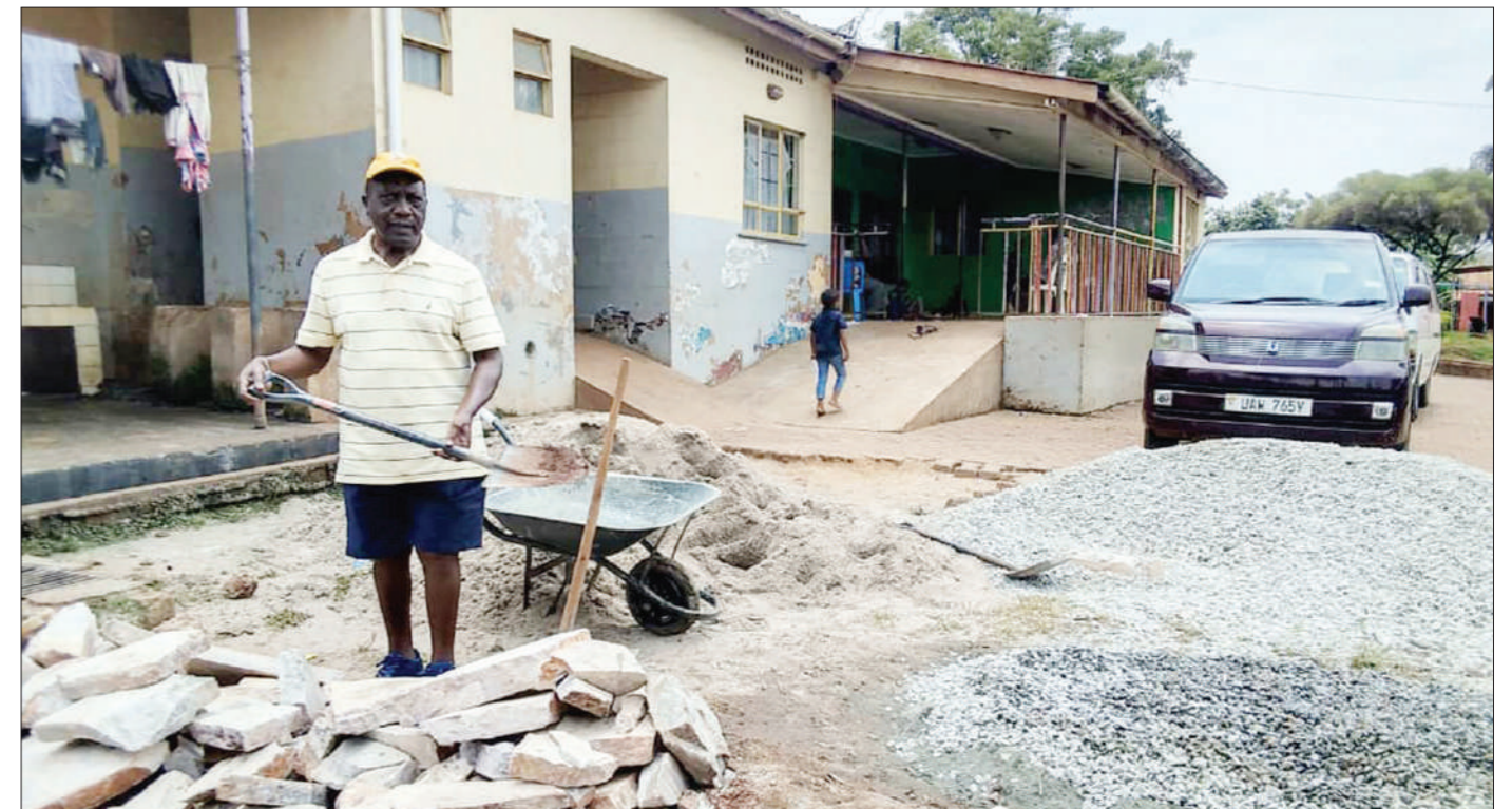
Renovation works by RC Kaolol-Kampala at the Naguru Children's Reception Centre
