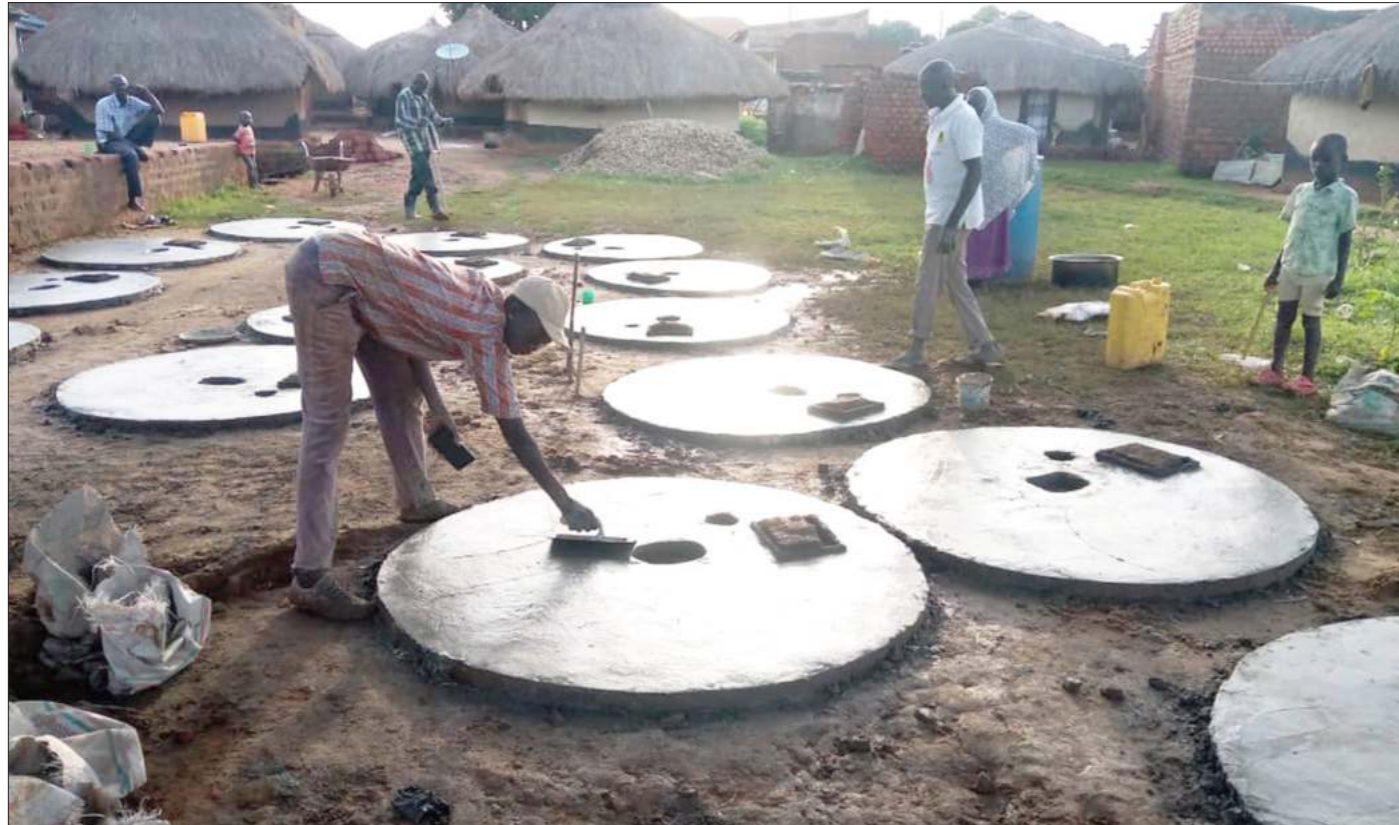
Beatrice demonstrating how to make latrine Coverplates in Injua village, Yumbe
