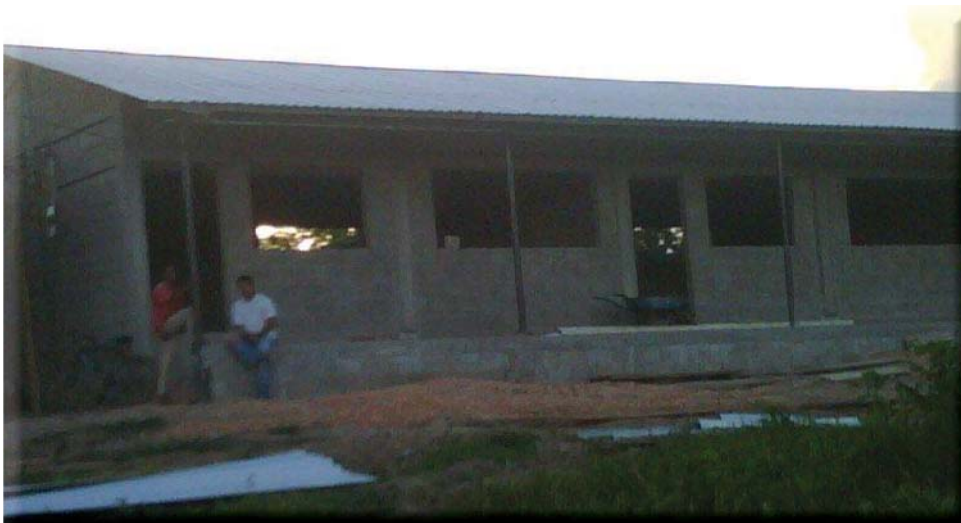
The new Las Lemus school nearing completion
