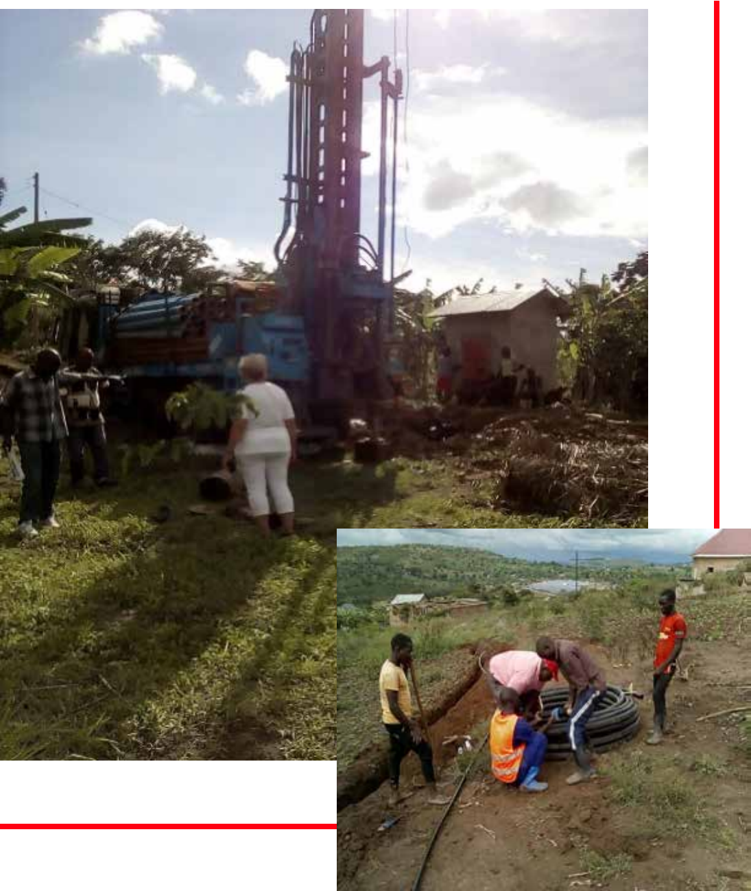
“The production well being drilled and pipe lines being connected to the well and reservoir”.
