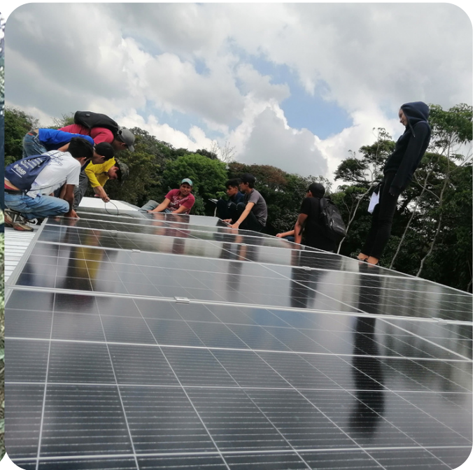
Installation of photovoltaic solar system, carried out by young students from the Rodeo community.
