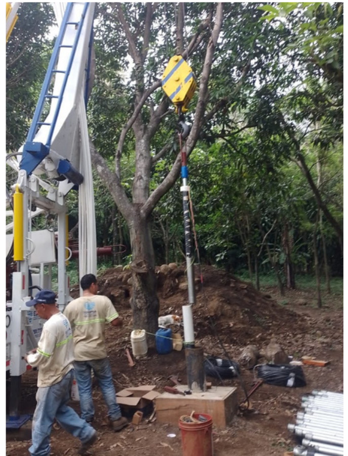
Pump installation inside the mechanical well.
