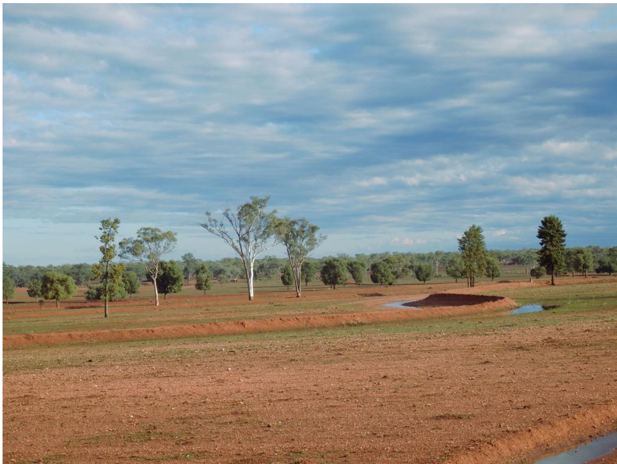
Our front paddock a few days after the 14.5mm – waterspreading banks assist in taking the energy out of the water so it has time to soak in, thereby in effect watering the paddock. Photo taken 17.10.18
