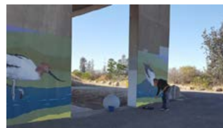
Scott Lewis applying anti graffiti coating
