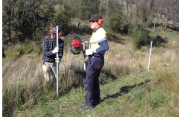
Using a dropper knocker to drive in a steel post on a fence, with the creek line behind at the bottom of the valley.
