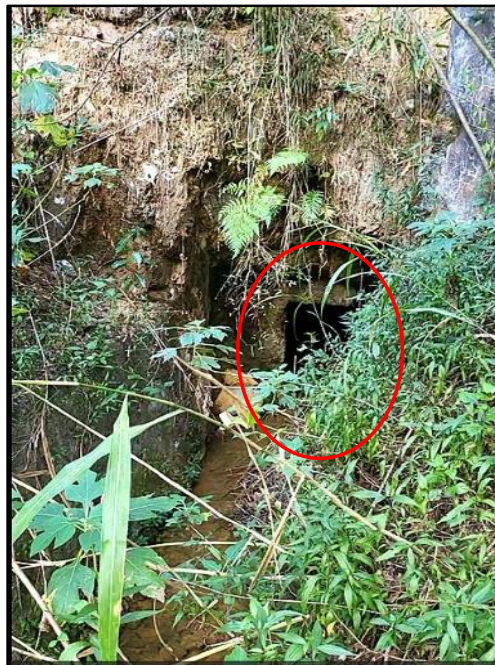
Figure 4 – This picture shows the mouth of the tunnel where the spring water comes out of.
