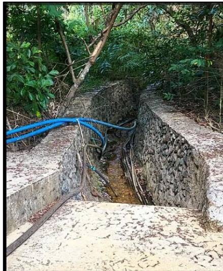
Figure 2 – This is the tail end of the concrete-lined canal which starts from the mouth of the tunnel. The flat concrete at the bottom of the picture is part of the unused water storage or holding tanks. Notice the flexible PVC pipes in the canal which were attempts by residents to tap the water for their individual household water supply.
