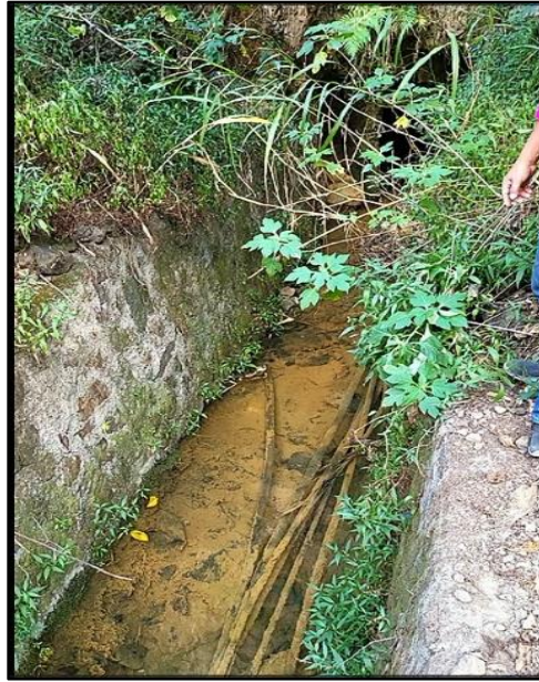
Figure 3 – A section of the concrete-lined canal with the clear flowing spring water.
