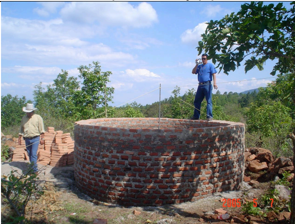
A water tank under construction
