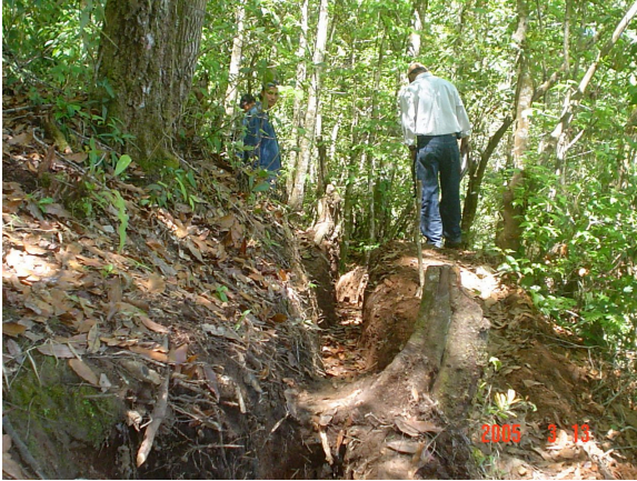
Manual labour required to lay pipe
